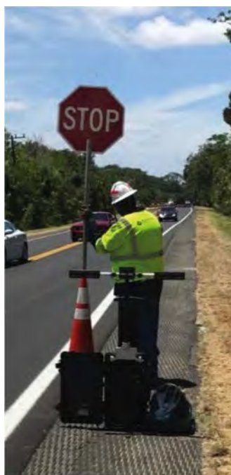
Figure 8. Self-contained intrusion alarm system for flagging operations (images courtesy of Oldcastle Materials).
