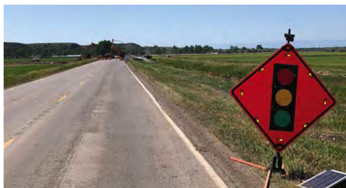
Figure 12. MDT warning sign with LED lights (image courtesy of Montana DOT).
