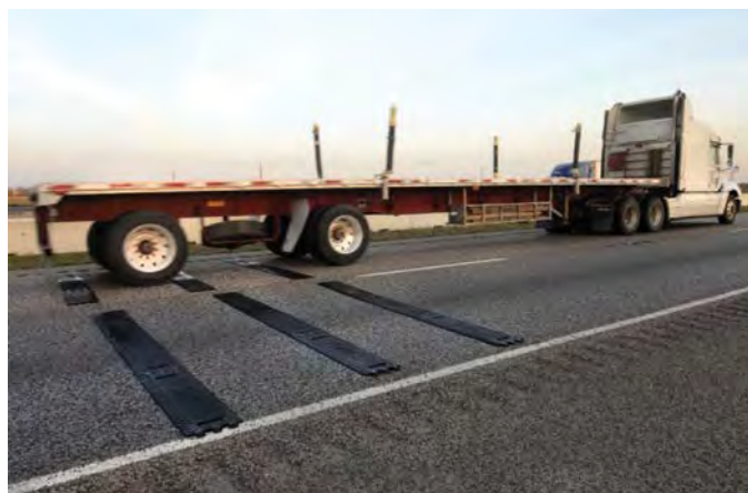
Figure 3. Example of TPRSs deployed upstream of an interstate lane closure (Ullman et al. 2018b).
