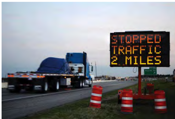
Figure 2. Example of work-zone ITS queue warning technology (Ullman et al. 2016a).
